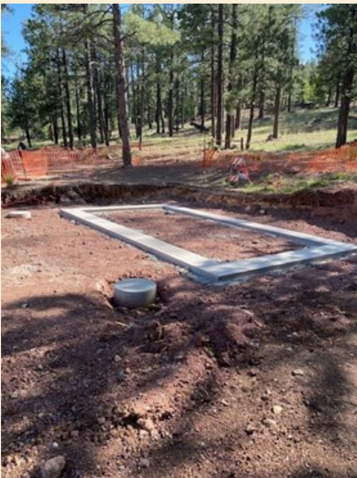
Foundation for the Thorpe Park Restroom
