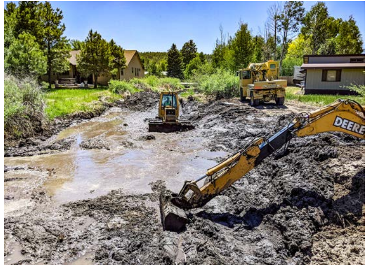
Open channel maintenance.
