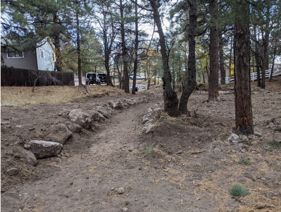
Figure 5. Repaired Fanning Wash channel upstream of Steve's Blvd following flooding, note new rock lined channel and the removal of debris on the right flood terrace.
