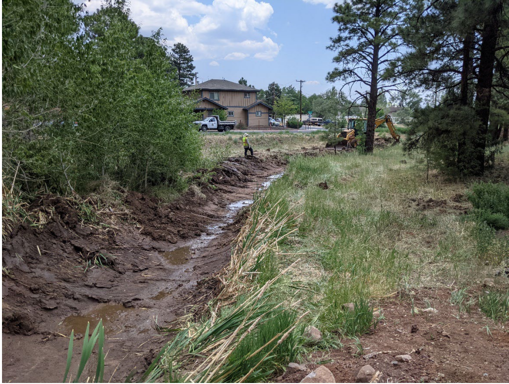
Figure 6. West Wash dredging by Water Sewer Collections crew near Izabel and Colanthe Streets.
