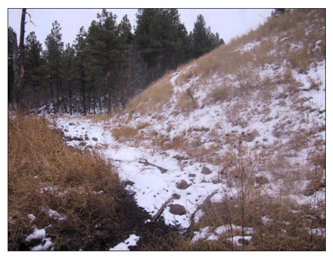
Figure A6. Steep road embankment at "C" adds excessive sediment to stream channel.
