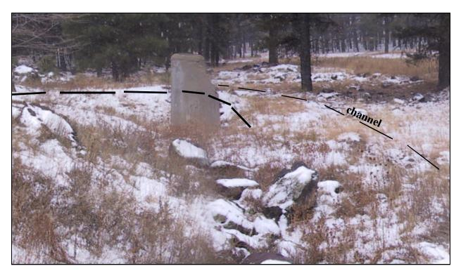
Figure A8. Existing manhole lies exposed in floodplain. Left terrace will be extended to include manhole to improve aesthetics and reduce floodplain scour. Area "N" on site map.
