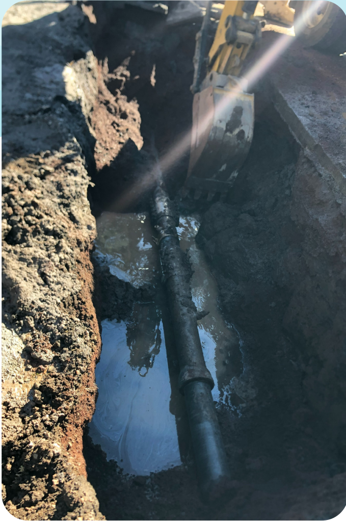
Emergency crews excavated and repaired several breaks along a 1962 6" cast iron main on Silver Spruce Ave.
