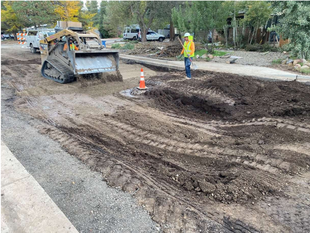
Talkington/Louise intersection, looking north at subgrade stabilization
