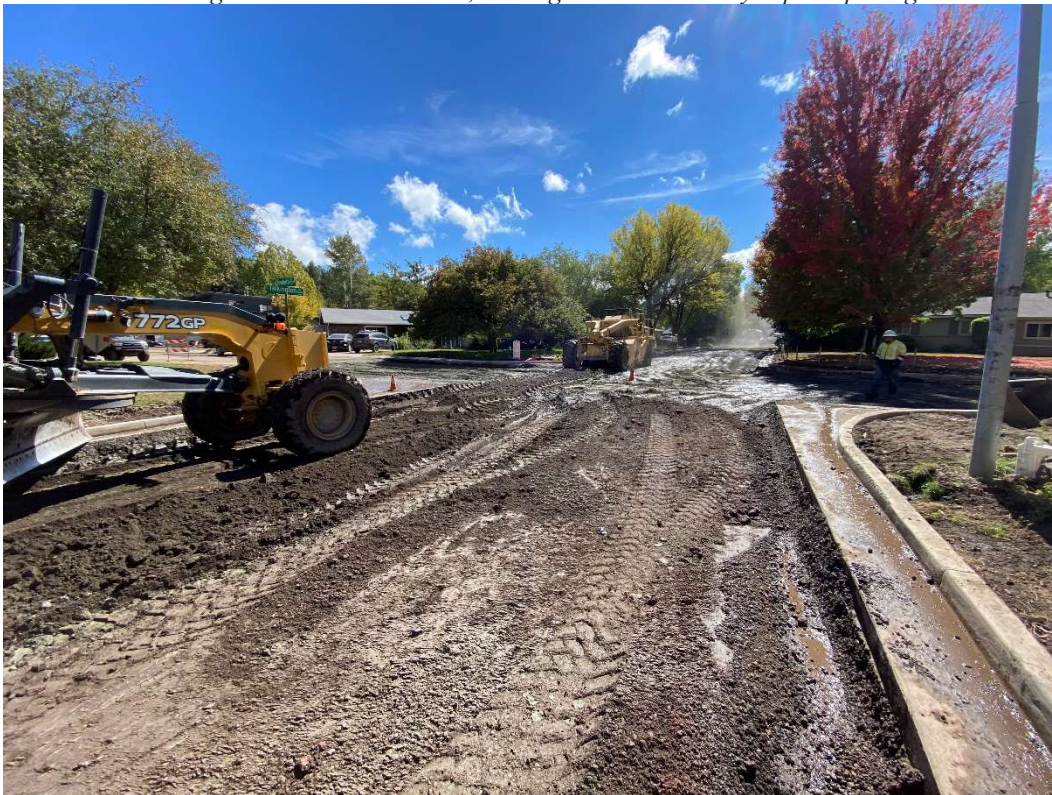
Talkington/Elizabeth intersection, looking south at subgrade stabilization
