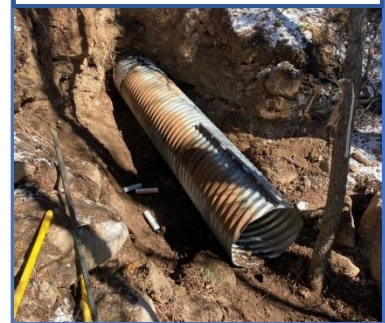
12" stormwater pipe extended on Appalachian Way
