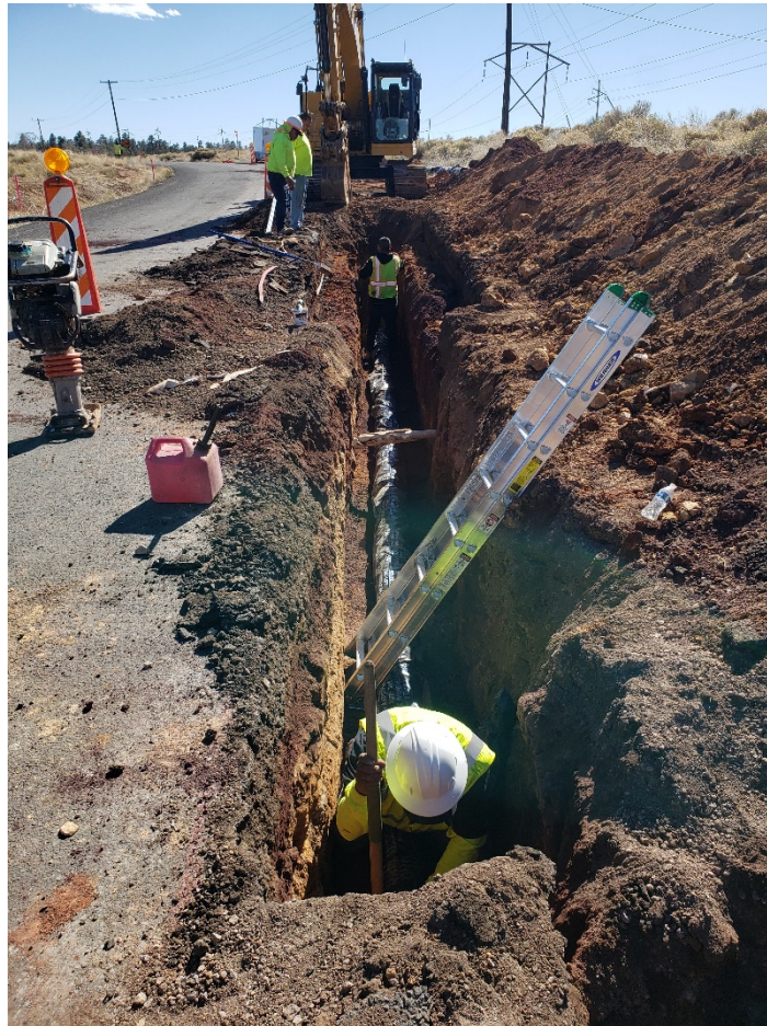
El Paso Flagstaff Rd., looking south at the start of the installation of the 8” ductile iron waterline
