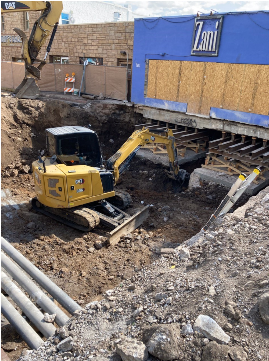
Phoenix Avenue Bridge, looking south at completed demolition and start of soil excavation to bedrock
