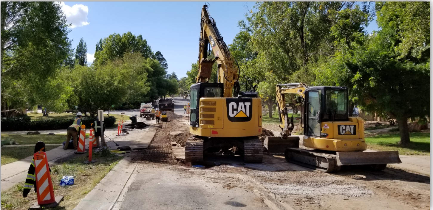
Beal Rd. west of Rio de Flag, looking west at water main and service installations.
