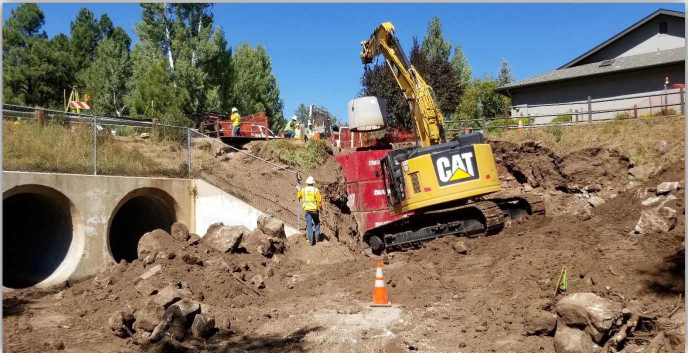
Crescent Dr. and Rio de Flag, looking north at the new sewer main installations connecting Crescent and Rio de Flag sewer mains.
