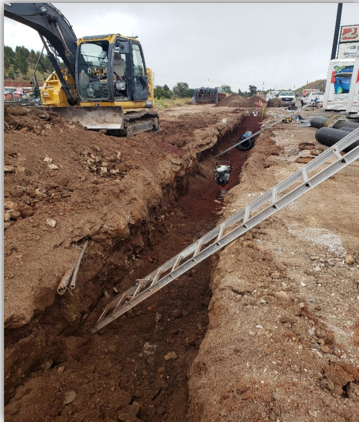
Installation of the 16" waterline
