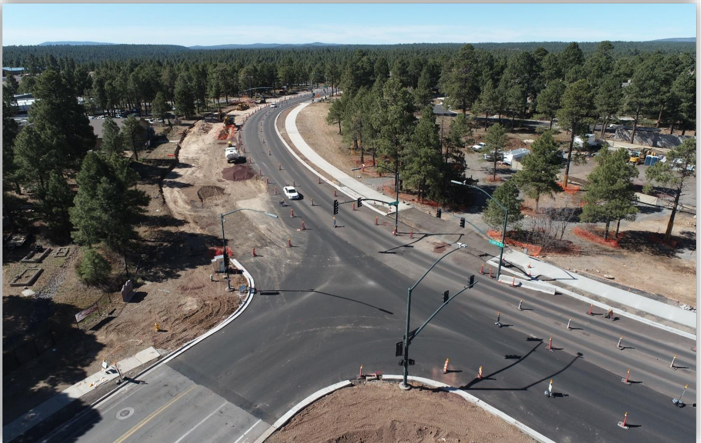
Fourth Street Reconstruction –Soliere Ave. base lift paved and reopened
