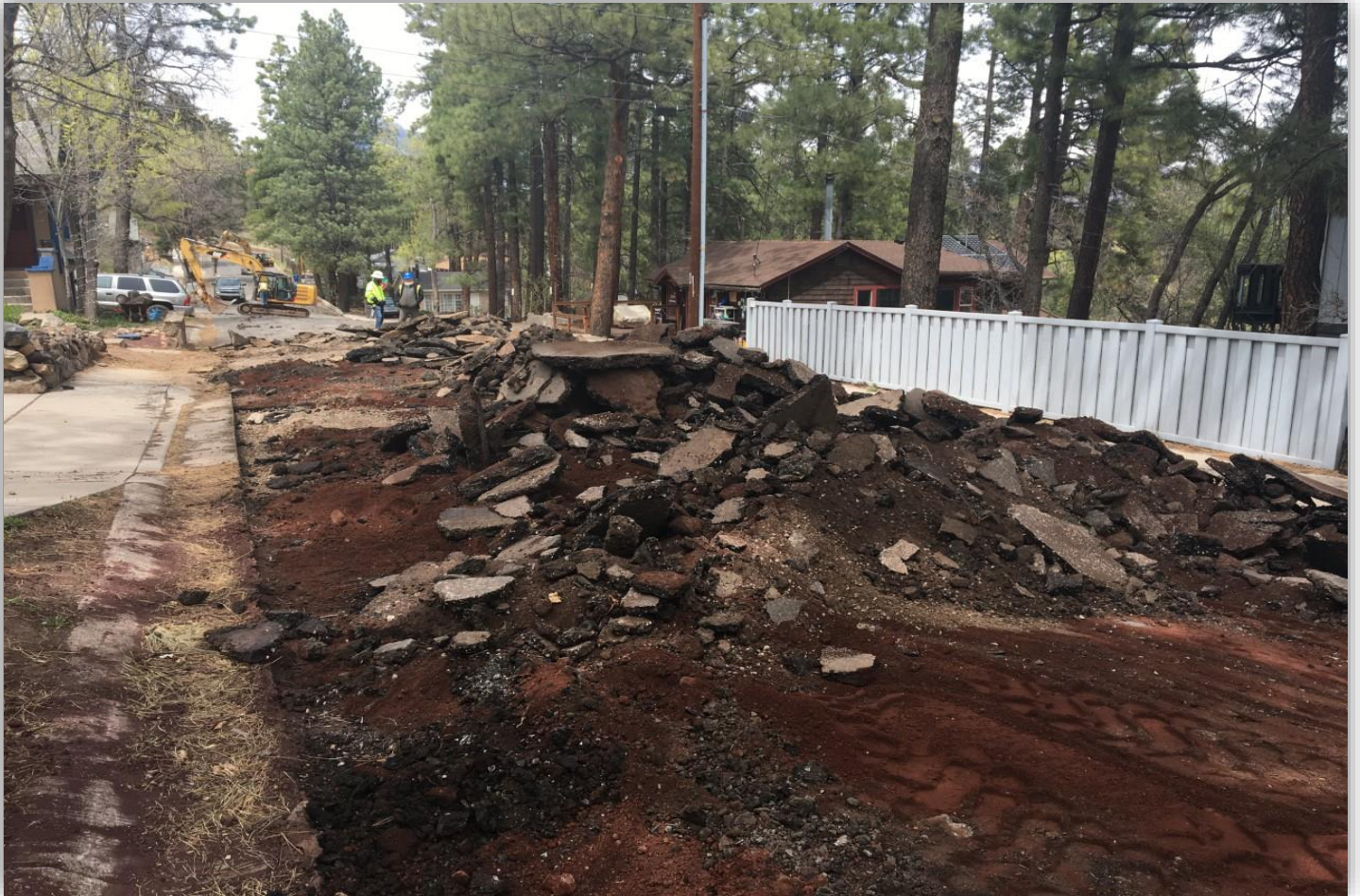
Summit Water Project-Spring St. pavement removal
