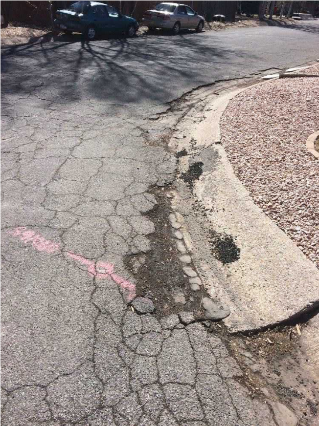
Photo No. 1: Alligator cracking, corner erosion and Asphalt spalling on N. Navajo Drive
