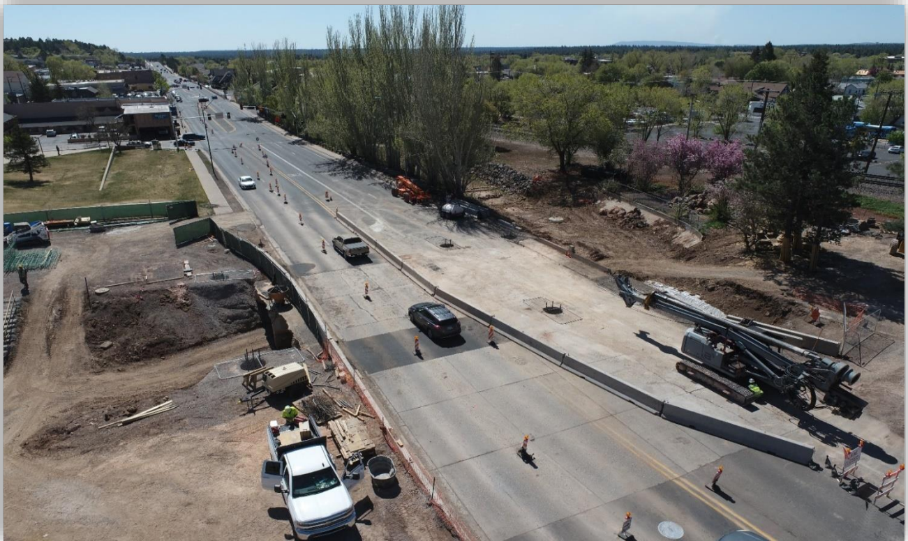
Equipment on site for the drilled shafts. Work performed on south side of Rt. 66
