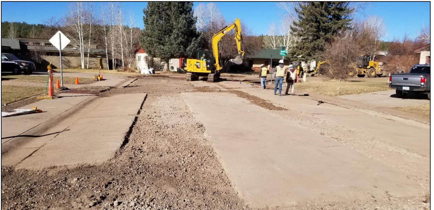
Navajo Rd. / Navajo Dr. intersection looking west Preparing the roadway for asphalt patching over trenches for a clean site prior to the Neighborhood Luminarias Event
