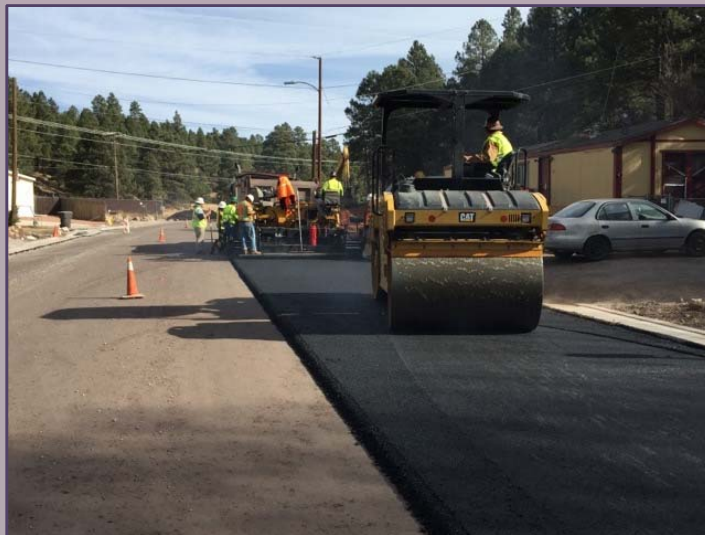
Zuni Drive Improvements
