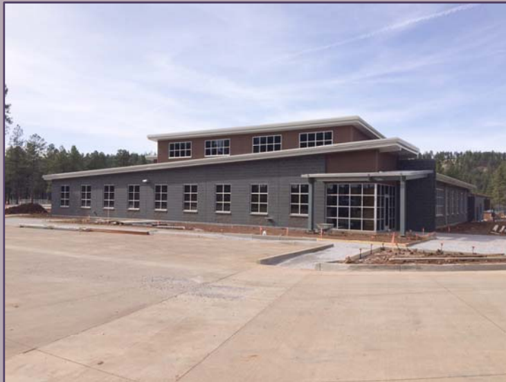
Core Services Maintenance Facility
