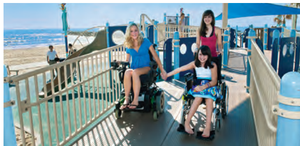
This double-wide ramp exceeds ADAAG standards to offer more size and space for approach and use while also providing an alternative route for play.
