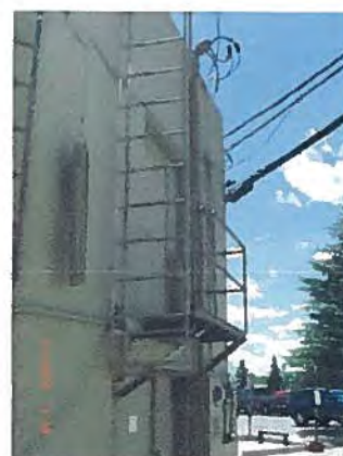
Photograph 24. Fire escape with pull down ladder, 2 nd floor balcony, and first floor door – southwest corner of building.
