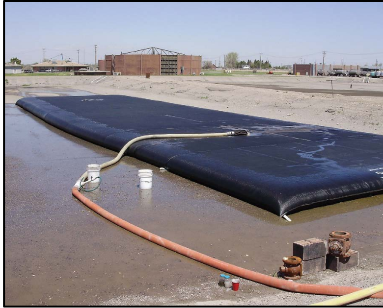
Figure 6 Geotube® Container on Lay Down Area
