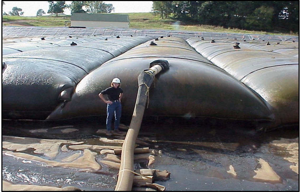
Figure 8 Geotube® Dewatering
